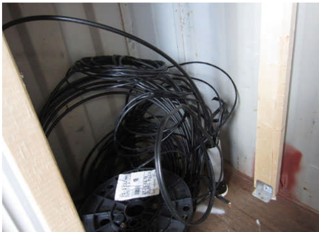
the original cables inside the Support Building
